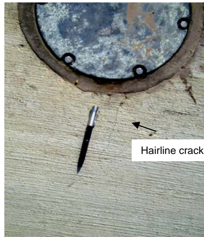
Figure 7.3 - Early Cracking in Pavement
