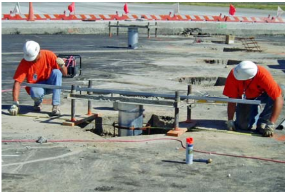
Figure A.4 - Setting the Light Base Using a Jig.
