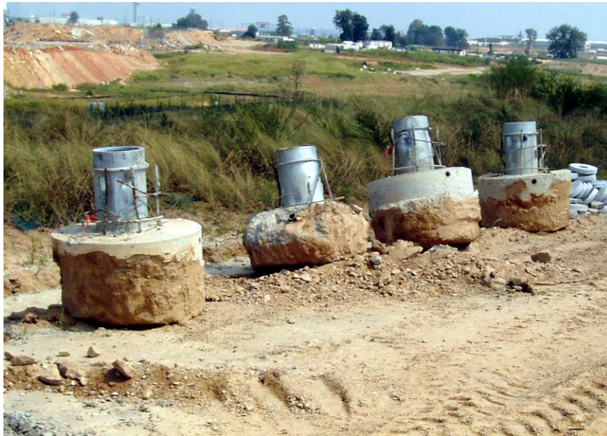
Figure 7.1 - Fate of Deficient Light Base Installation.
