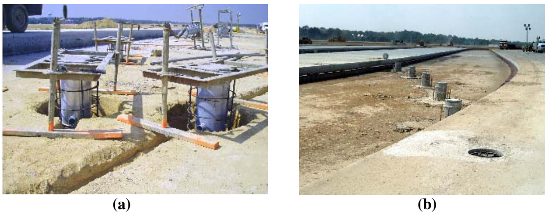
Figure 4.1 - Taxiway Centerline Light Base Installation at Intersecting Taxiways.
